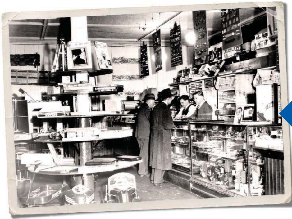
Sager Electrical Supply, Congress St., Boston, MA.
