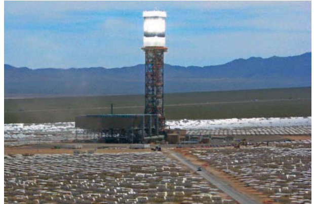
IoT Technologies can coordinate the rotation of the hundreds of thousands of mirrors to maximize energy production at the Ivanpah Solar Electric Generating System on the California-Nevada border. (courtesy of Business Wire)
